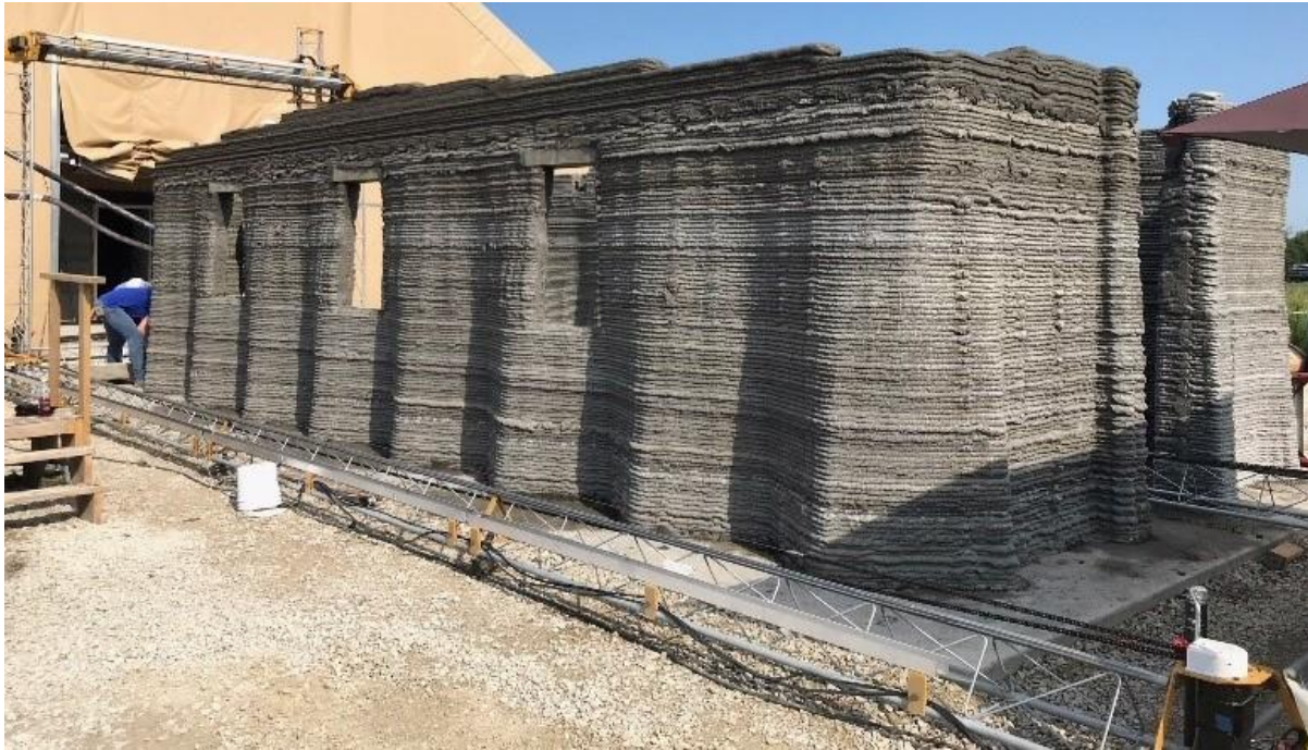
Figure 20 – 3D printing a building
